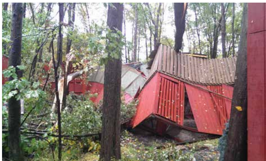
Large flight cage number one, completely destroyed.
